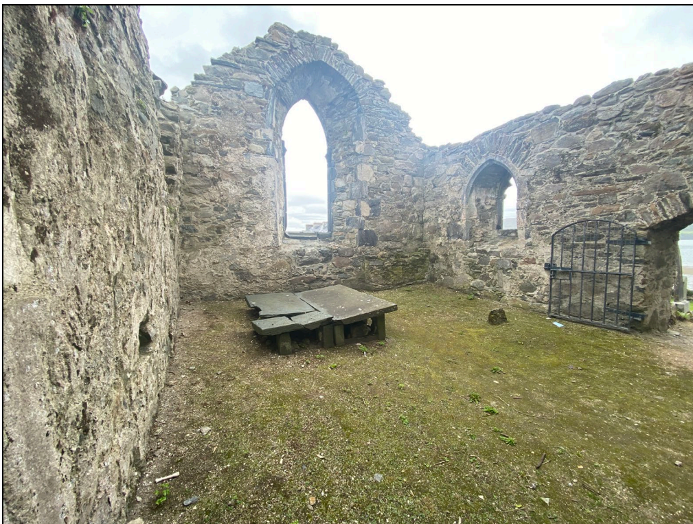
Plate 11: East facing view of the Chancel.
