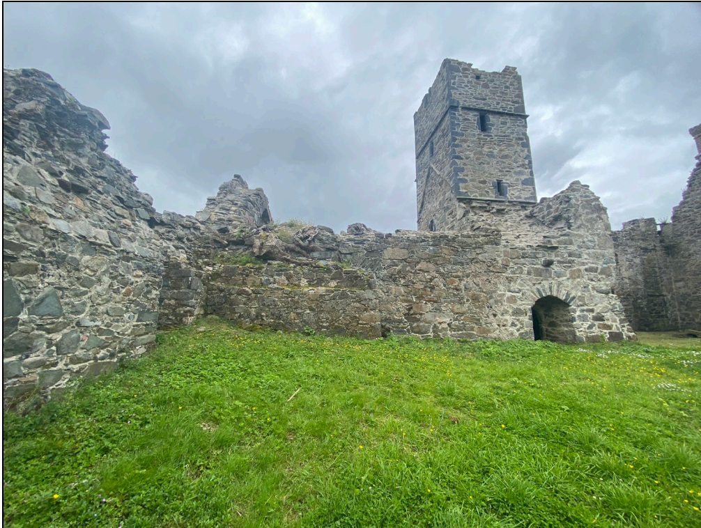
Plate 14: South facing view from the cloister area looking towards the tower.
