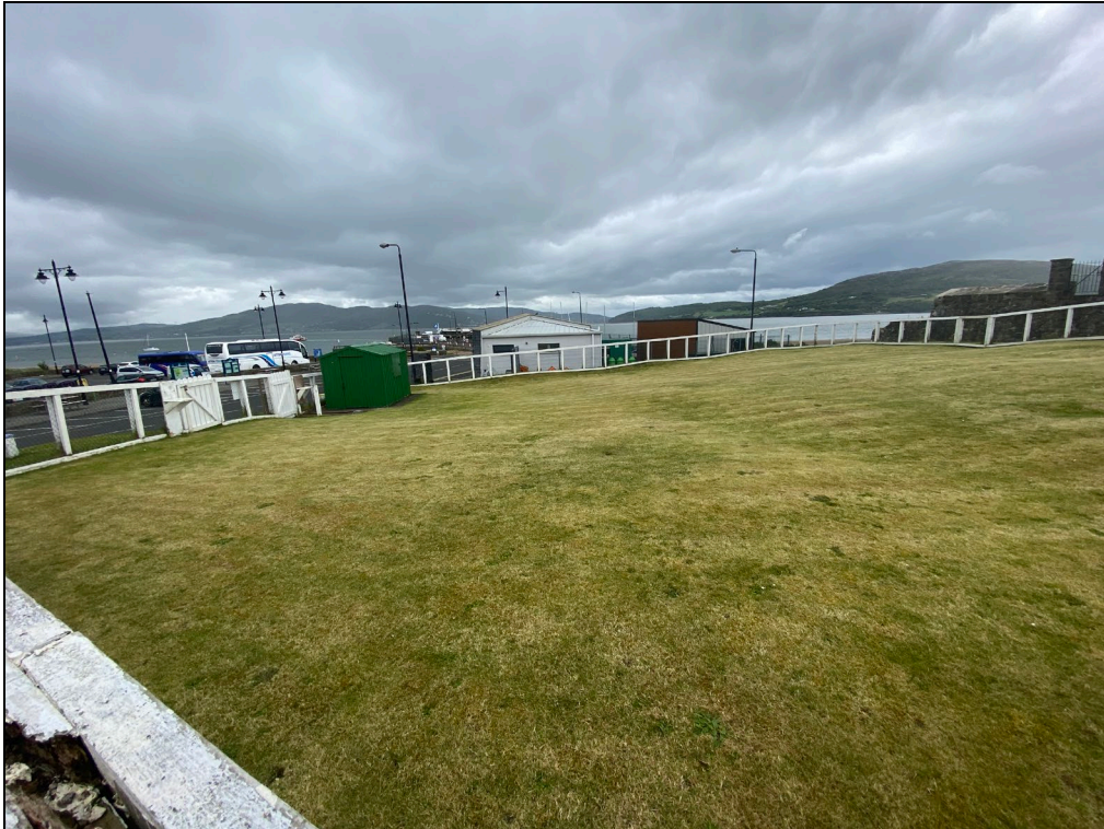
Plate 5: South facing view of the Glacis through which a footpath is proposed.
