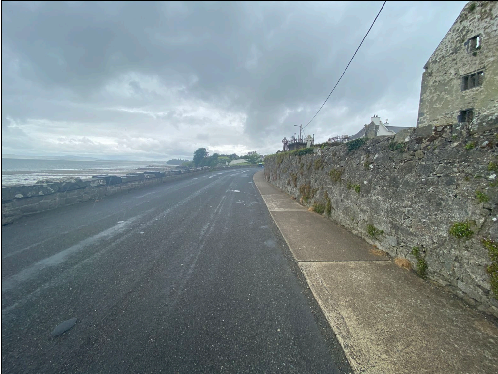
Plate 18: West facing view of Main Street with the Abbey visible to the right.
