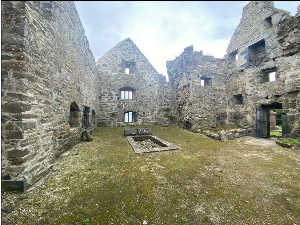
Plate 10: South facing view of the Transept.
